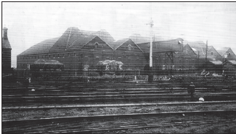
Figure 4 Dereham railway station (1921) showing extensive maltings (built 1850) and waggons loaded with sacked barley or malt
