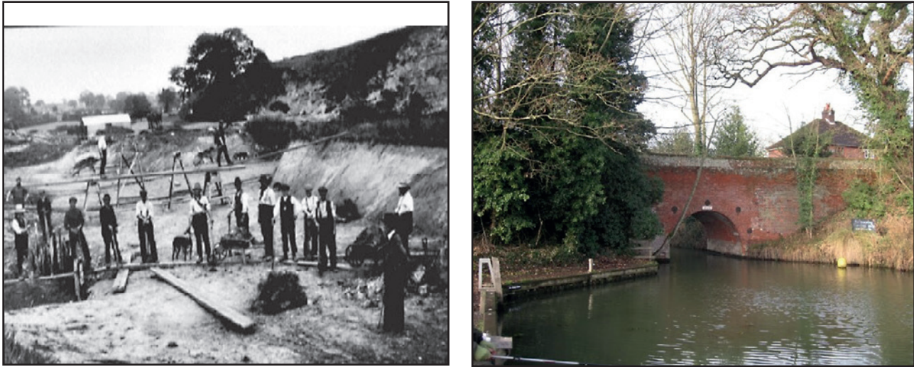
Figure 3 The construction of North Walsham and Dilham Canal (1825-1826) [1] and 'Tyler's Cut' connecting Thomas Taylor's brickyard to the Canal [r]
