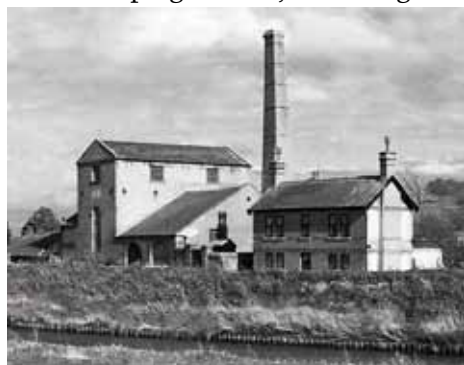
Stretham Engine House, near Ely
