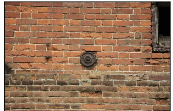
*P5 - Above: Detail of North elevation wall brickwork and tie plate*
